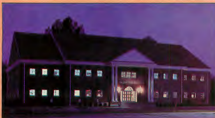
Located just outside of Louisville, Kentucky, in the small town of Prospect, the Falsoft Building is, indeed, the house that RAINBOW built.
