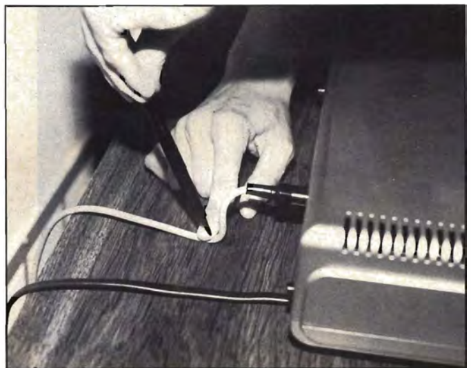
Photo 2. Do not force cables to bend too sharply.
