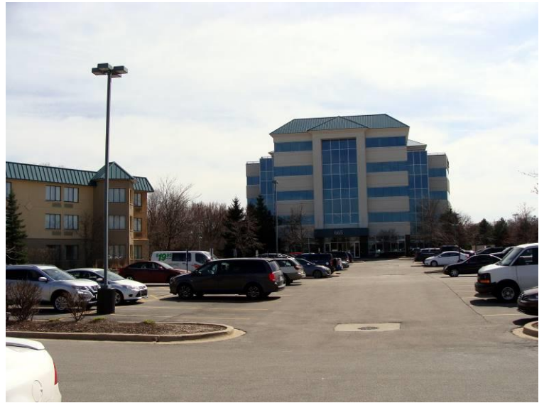
The Inn is on the left and the Heron Point Building is on the right
