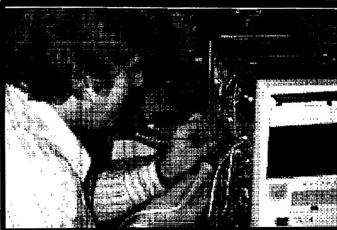
*Mark Kulien* installing an internal Modem to Donald Zimmerman's CoCo-3 in PC Tower Case
