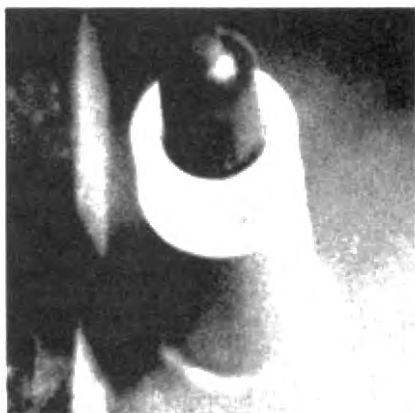
Photo 5. Grommets installed on the left and right support posts.
